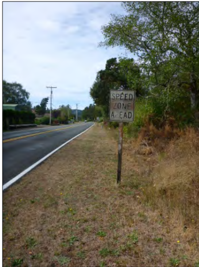
Old Tokeland Rd Route 9513 – Faded, rusted sign. (Photo #169)
