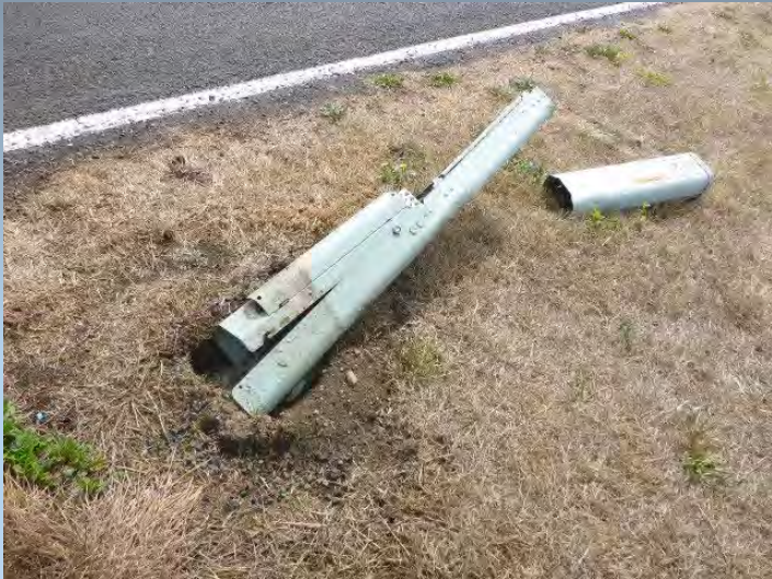
Route 9995 - Kindred Ave #279
