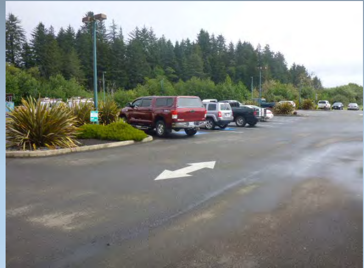
Route 0308 Casino Parking Lot #100
