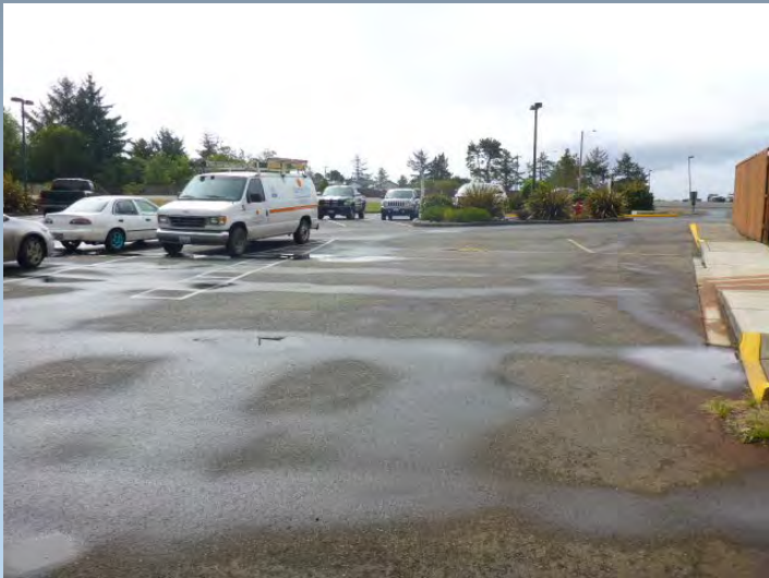
Route 0308 Casino Parking Lot #111
