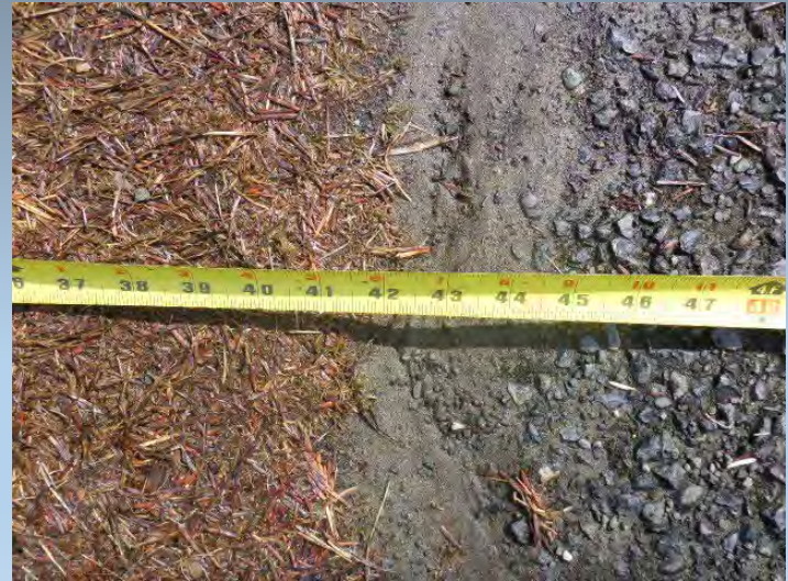
Route 9990 Site Deficiency #276
