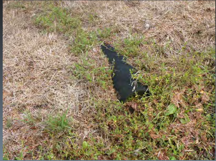
Route 9513 Buried Culvert #237
