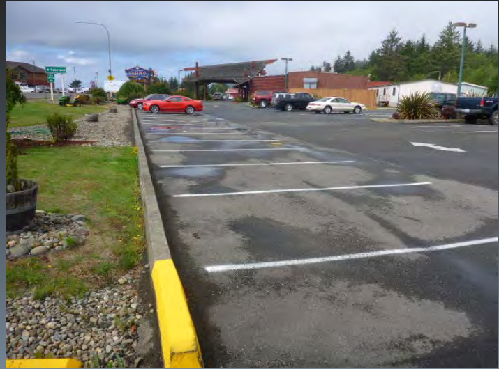
Route 0308 Casino Parking Lot #102
