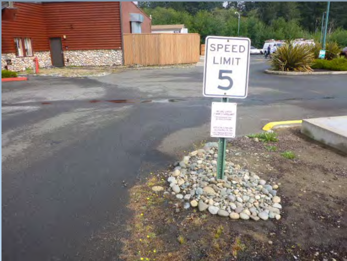
Route 0308 Casino Speed Limit Sign #135
