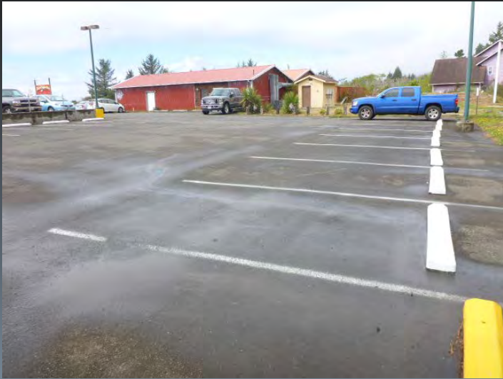
Route 0308 Casino Parking Lot #121
