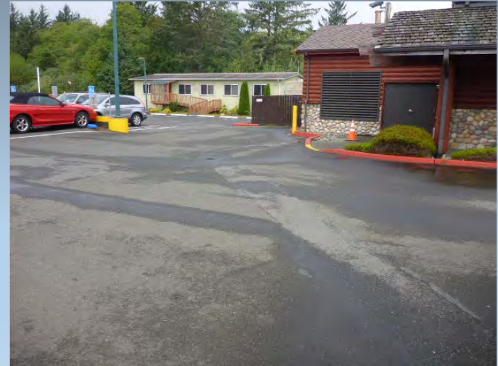
Route 0308 Casino Parking Lot #116
