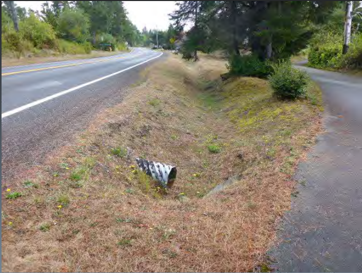
Route 0010 (Culvert to Culvert Connection) #29
