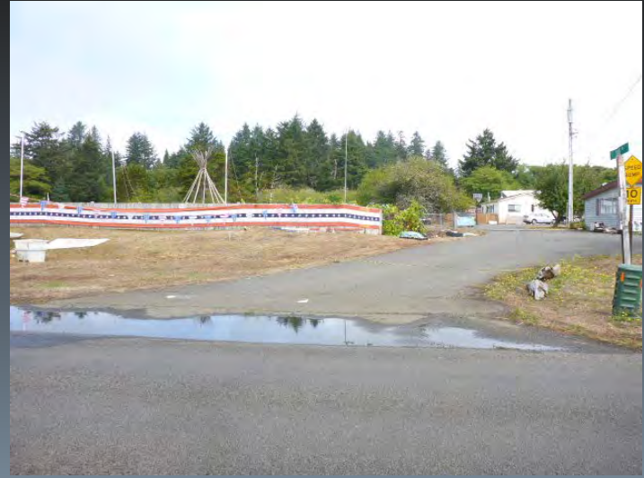
Route 9513 @ Route 9994 (Drainage Issues) #217
