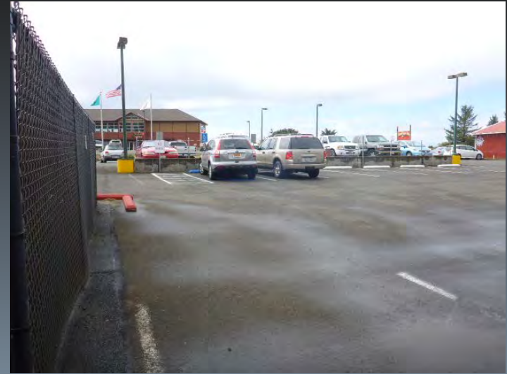
Route 0308 Casino Parking Lot #122
