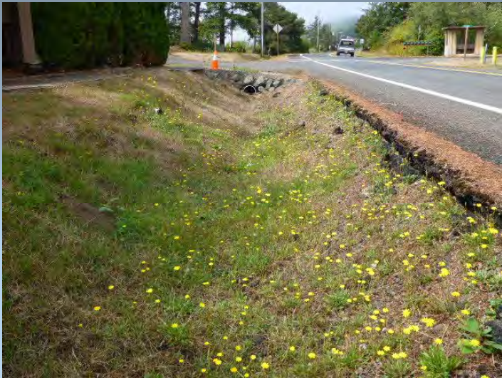
Route 9513 Drainage Ditch #246
