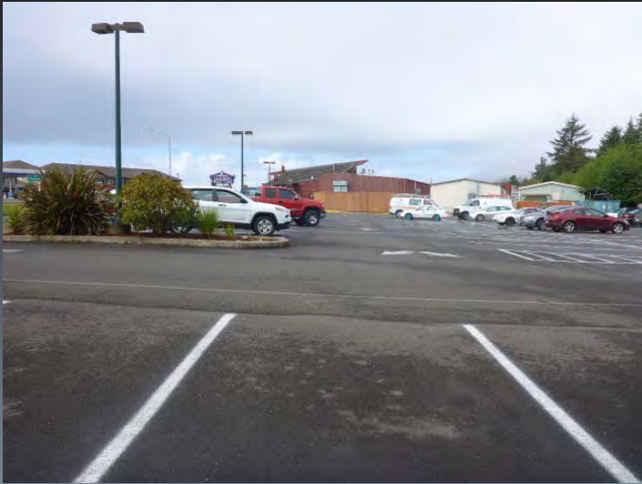
Route 0308 Casino Parking Lot #105
