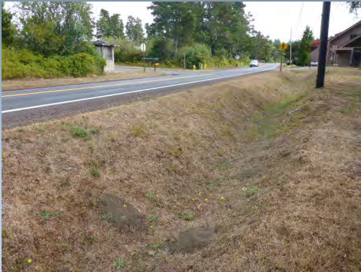
Route 9513 Drainage Ditch #242
