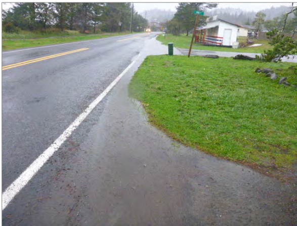
Old Tokeland Rd Route 9513 – Intersection with Davis Drive St – Route 9994 – Standing water – no ditch forces pedestrians into roadway. (Photo #156)
