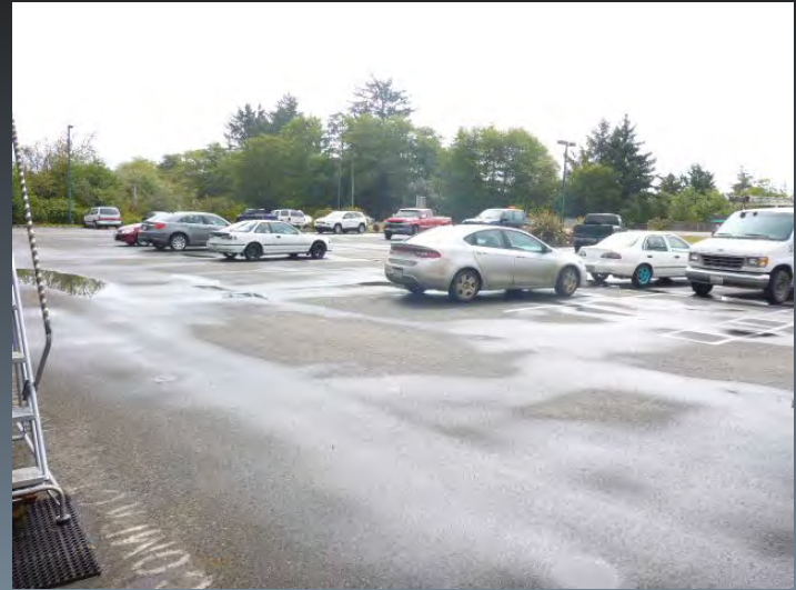
Route 0308 Casino Parking Lot #110
