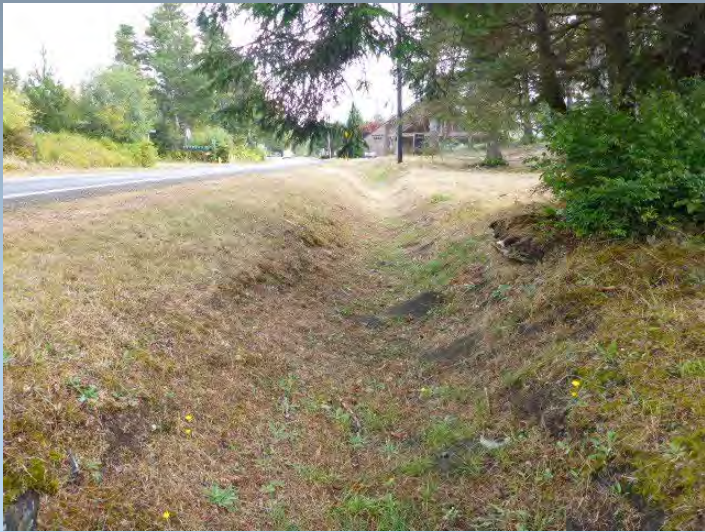
Route 9513 Drainage Ditch #250
