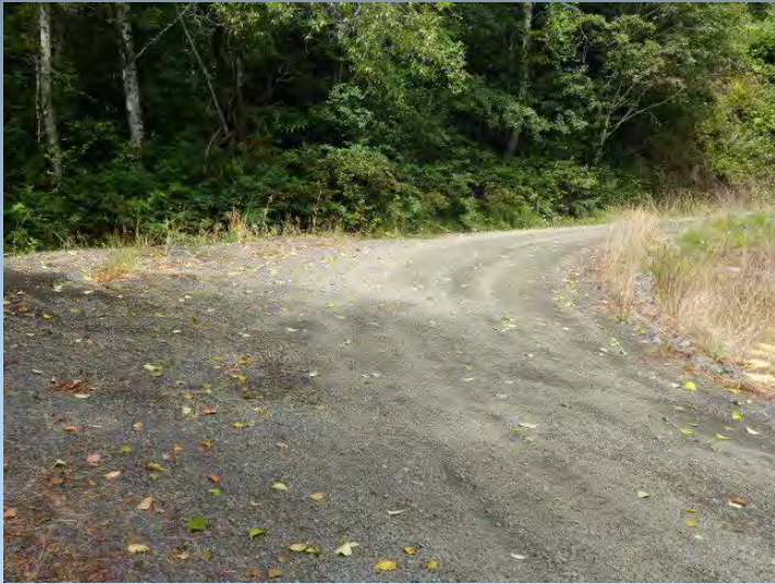
Route 0003 Road Curve #15
