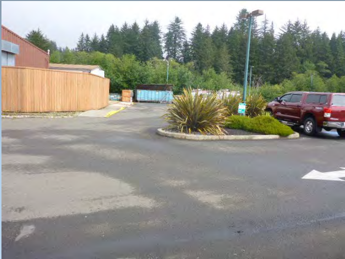
Route 0308 Casino Parking Lot #99
