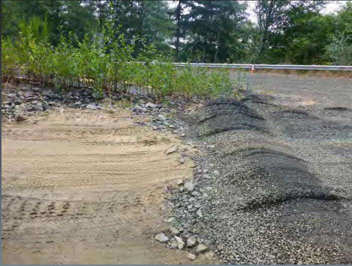
Route 0003 New Building Erosion Control #13
