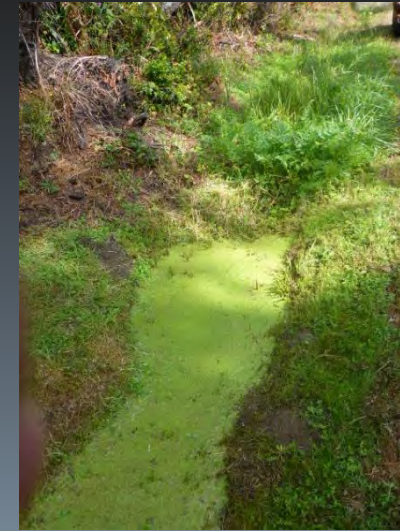
Route 0028 Drainage Issues #78
