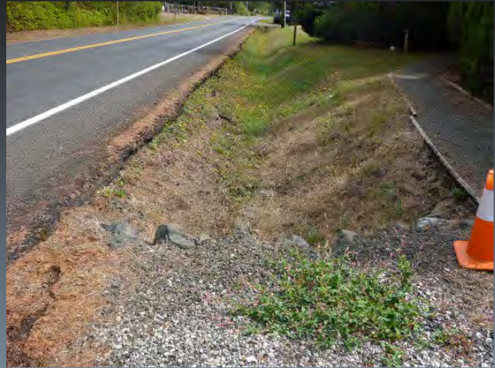
Route 9513 Drainage Ditch #245
