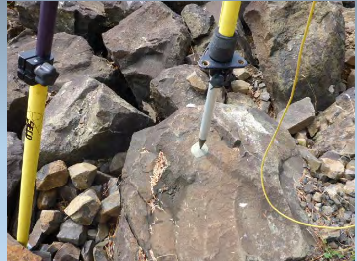
Route 0010 (Surveying Being Done) #44
