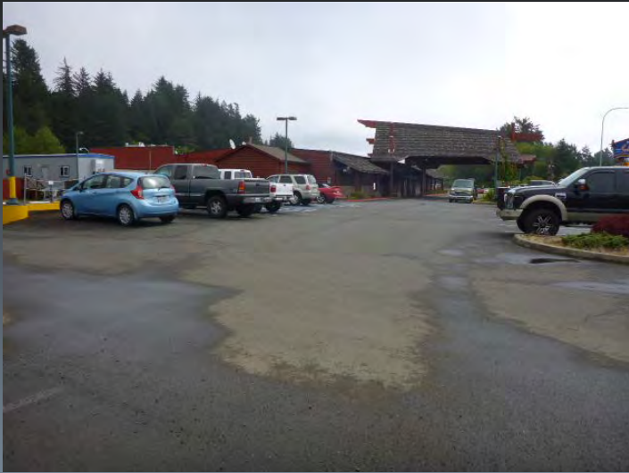
Route 0308 Casino Parking Lot #117
