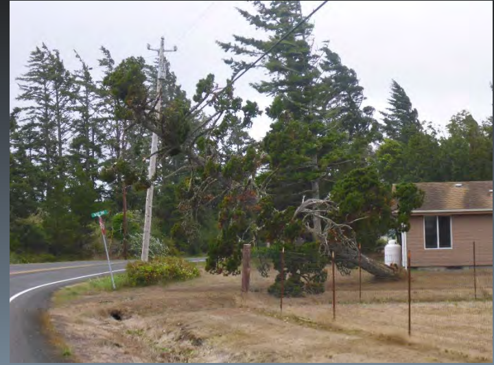
Tree on utility lines #326
