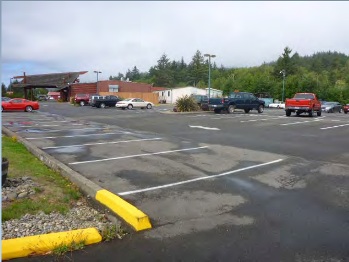
Route 0308 Casino Parking Lot #103
