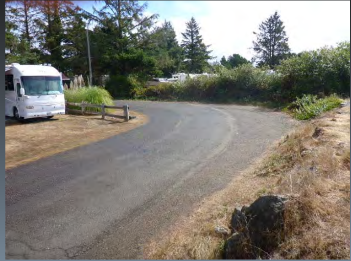
Route 9990 Site Deficiency #274
