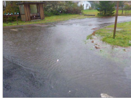
Old Tokeland Rd Route 9513 - Intersection with Georgetown St Route 0002. (Photo #148)
