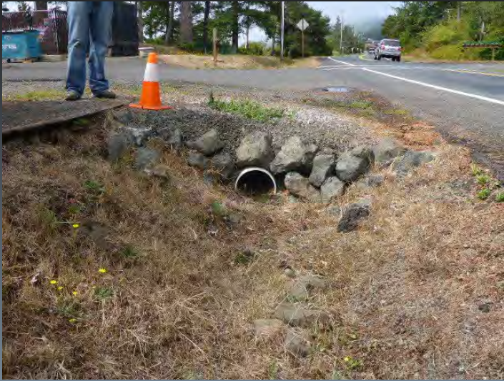
Route 9513 Drainage Ditch @ Culvert #248
