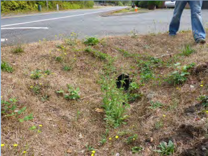
Route 9513 Ditch Culvert #238
