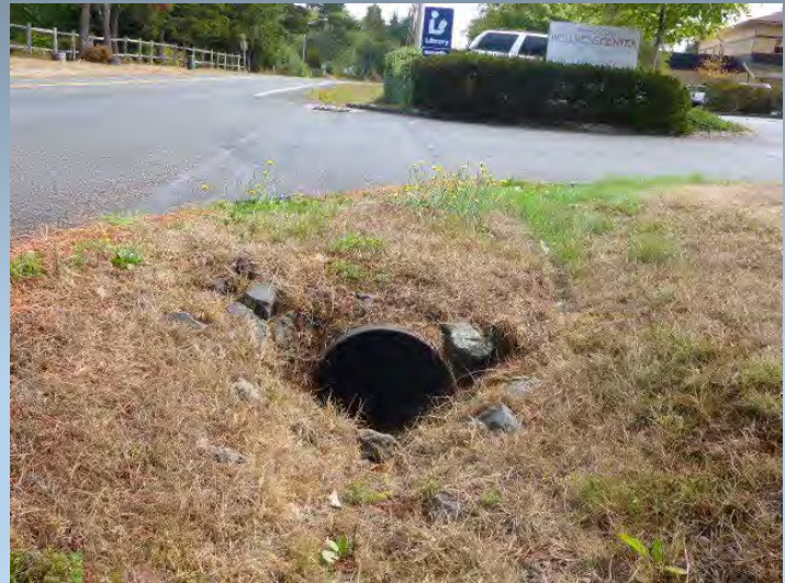
Route 9513 Drainage Ditch @ Culvert #247
