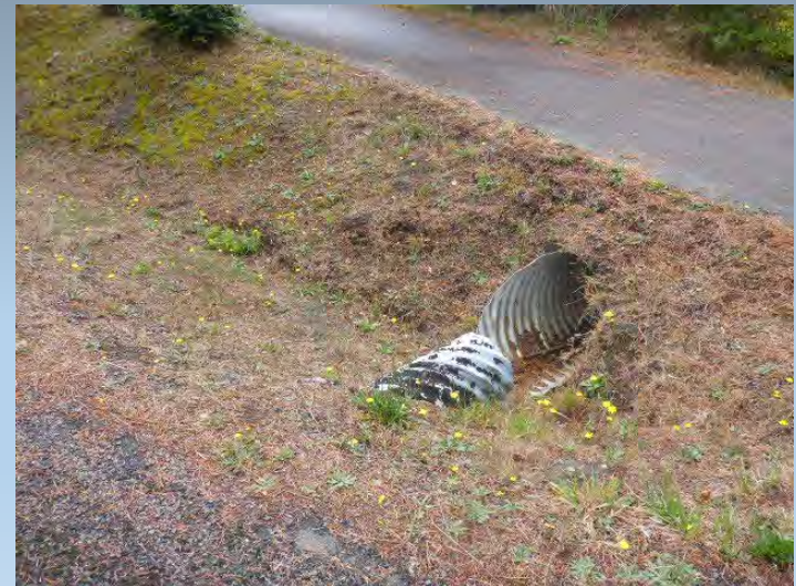
Route 0010 (Culvert to Culvert Connection) #28
