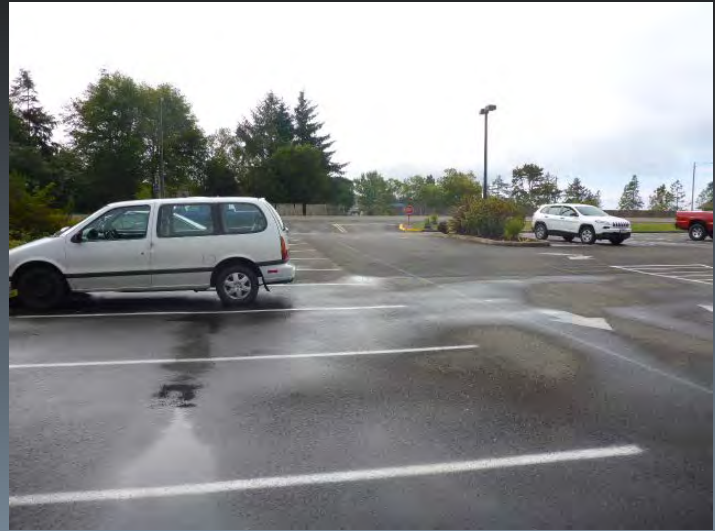
Route 0308 Casino Parking Lot #106
