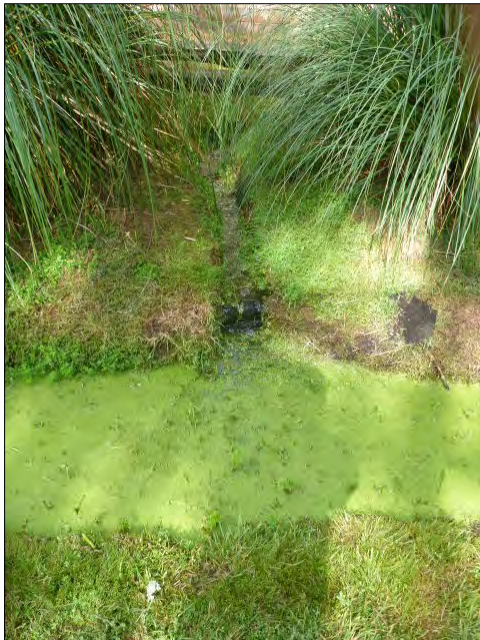
7 th St. Route 0028 – Plugged drain pipe. (Photo #77)
