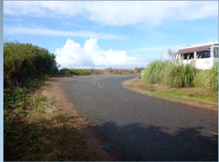
Route 9990 Site Deficiency #272
