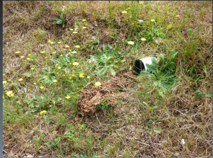
Route 9513 Drainage Ditch Culvert #249
