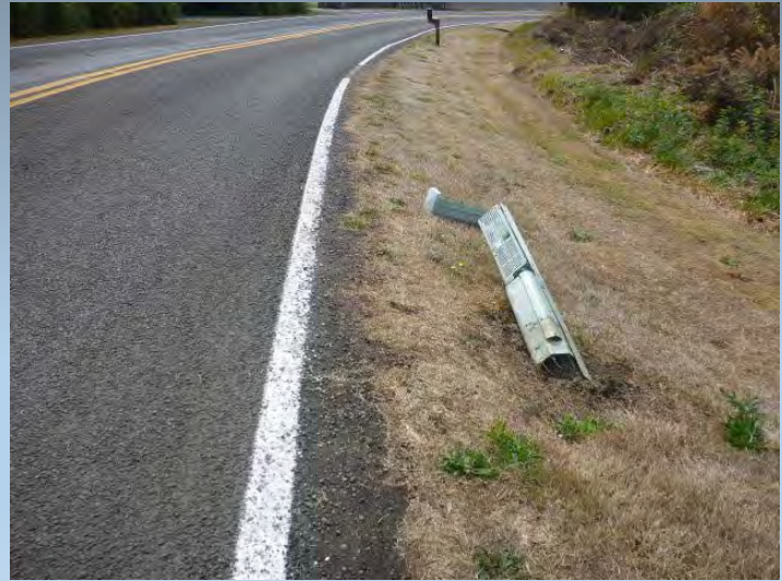
Route 9995 - Kindred Ave #284
