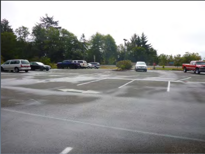
Route 0308 Casino Parking Lot #109
