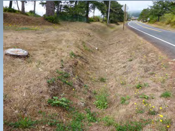
Route 9513 Drainage Ditch #243
