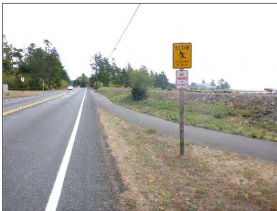
Pedestrian Trail Route 0010 – Pedestrian trail merges with Old Tokeland Rd. This creates a conflict between the pedestrians and cyclists and the traffic. (Photo #35)
