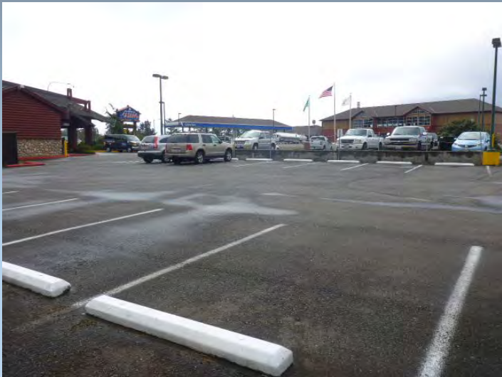
Route 0308 Casino Parking Lot #119
