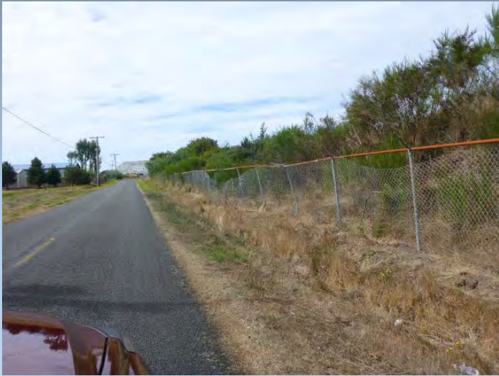
Route 9995 - Kindred Ave #283
