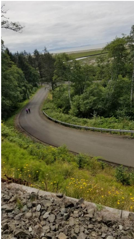
Figure 6: View from Eagle Hill Rd. from shelter
